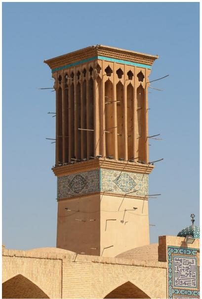
The wind catcher or wind tower is a traditional method to capture breezes to ventilate and cool houses> https://t.co/D8qg8ysaHf
